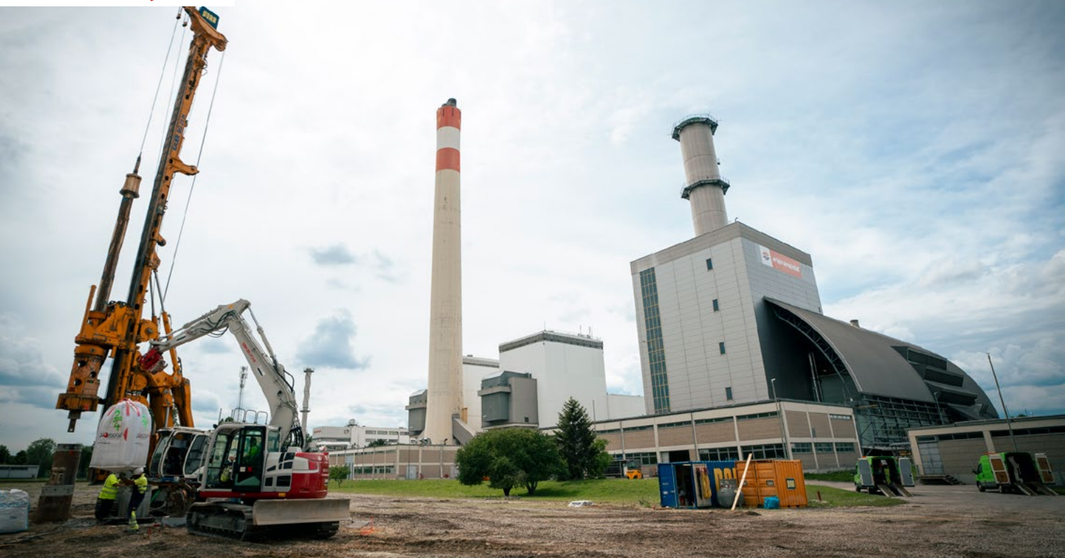
Drilling operations for the insulated bored pile retaining wall. Various materials are being tested for potential use in the future construction of the heat storage system. Photo: Wien Energie/ Michael Horak
