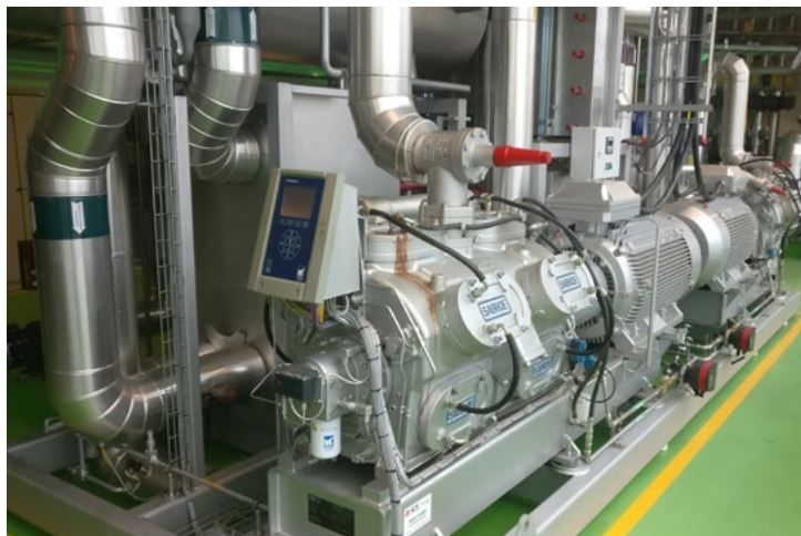
Heat pump for feeding waste heat into district heating networks, photo: 4ward Energy Research GmbH
