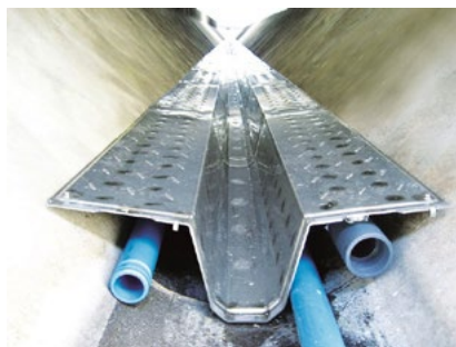
Heat exchanger in the sewer with dry weather channel, suitable from DIN 400, source: Rabmer Greentec GmbH, technology partner UHRIG
