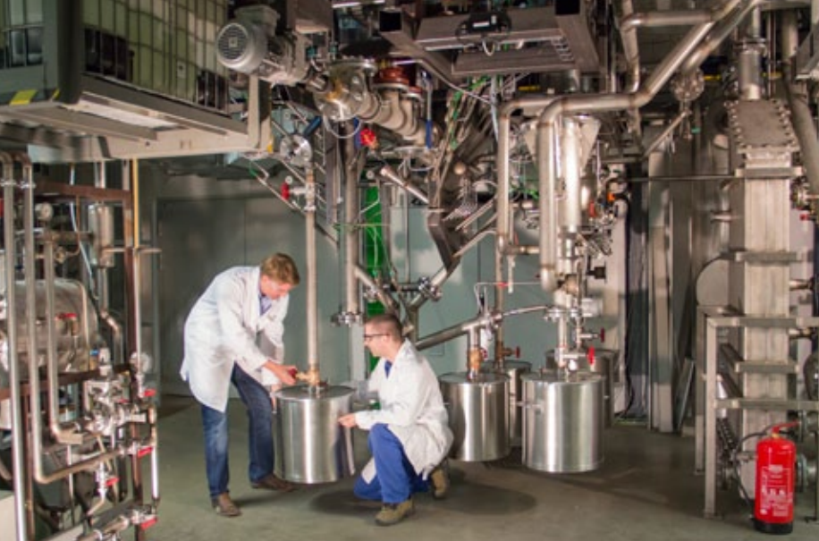
Lower part of the research plant without thermal insulation, photo: TU Wien
