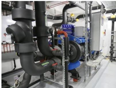
From left: server room as heat source, heat exchanger between server racks, pressure equalizer, chiller. Photos: Waldhör KG
