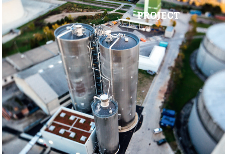
High-pressure heat storage facility at Simmering power station, source: Wien Energie/Ian Ehm
