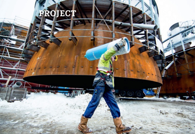
Construction of the high-pressure heat storage facility in progress, source: Wien Energie/Ian Ehm
