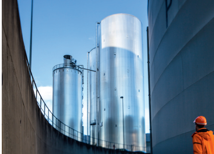
Heat storage facility, source: Wien Energie/Ian Ehm
