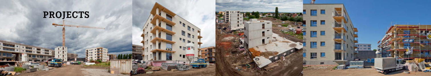
Phases of construction at surplus-energy cluster Reininghaus Süd, Source: Dipl.-Ing. Martin Grabner ECR-Team, Graz University of Technology, Institute of Urbanism
