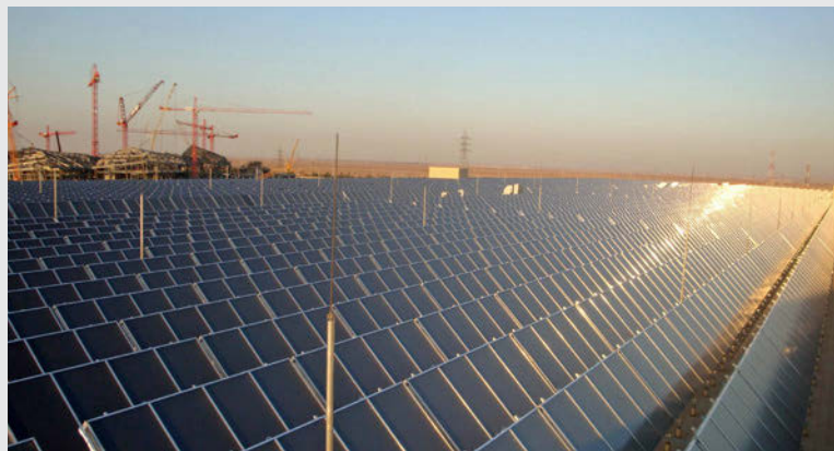
Photo: Millennium Energy Industries
